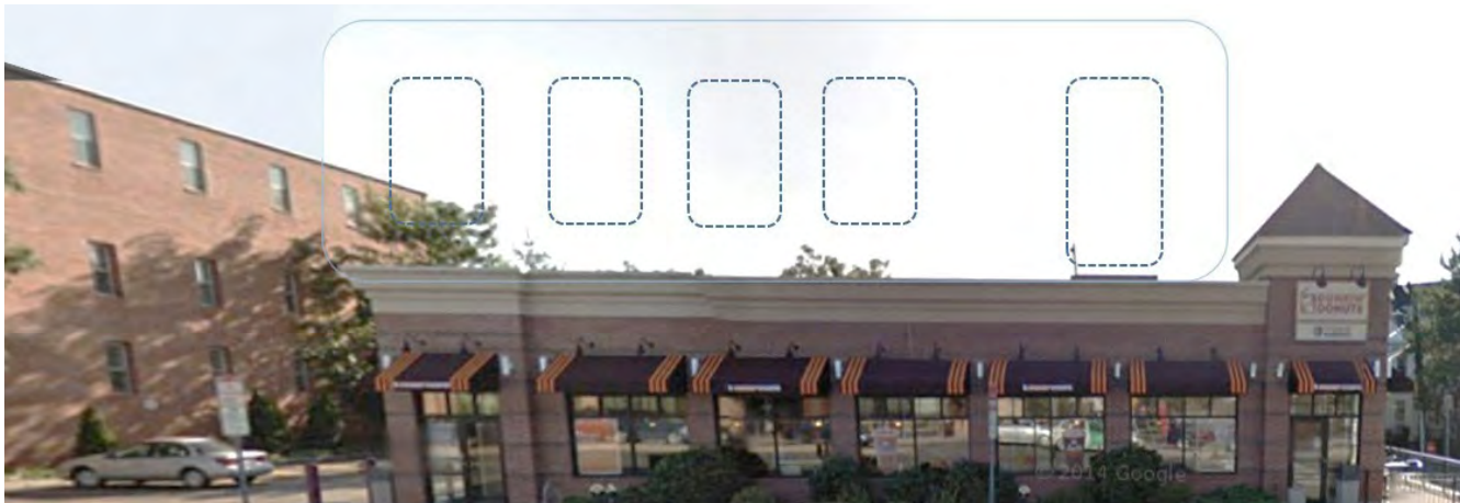
Figure 11: One story commercial building on Massachusetts Avenue, Cambridge, MA. Courtesy of google maps and the author.
