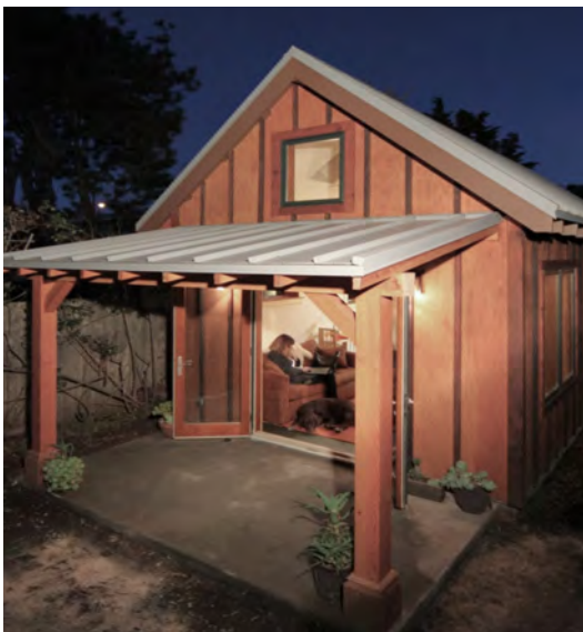
Figure 9 (Left): Completed accessory dwelling unit.
