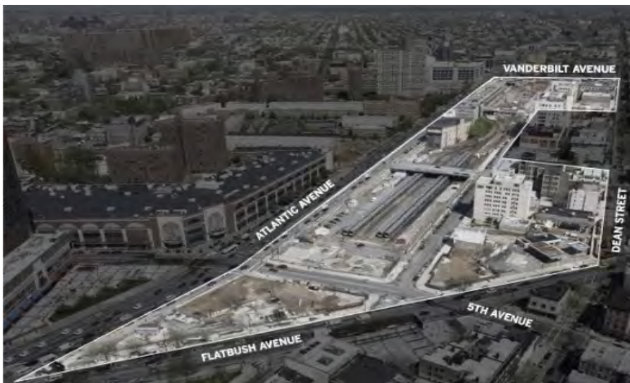
Image: Atlantic Yards (aka: Pacific Park Brooklyn). Image courtesy of the Bermingham Equipment Foundation.
